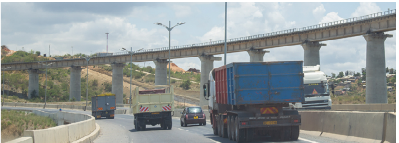
1st Phase of Dongo Kundu is completed and open to the public
