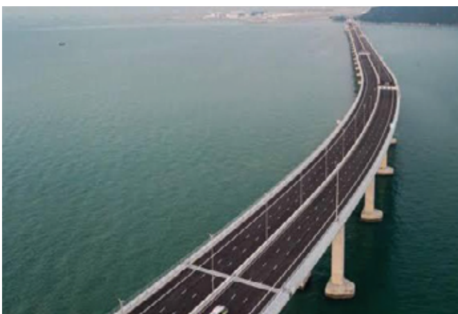
Second phase pillars for the bridge have already been erected.
