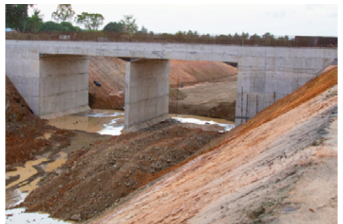
3rd phase is work in progress
